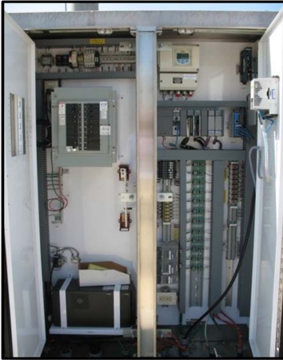
San Sevaine Turnout control panel
